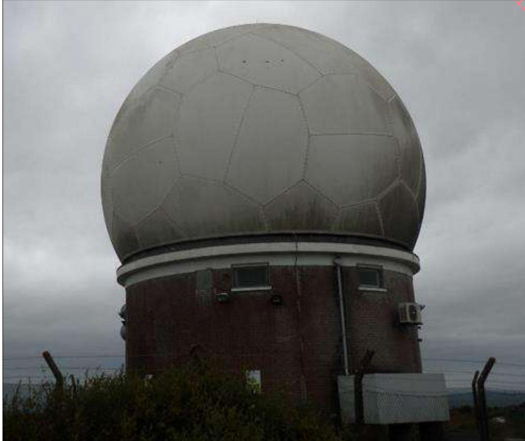
Figure 11. Woodcock Hill Radar Station
