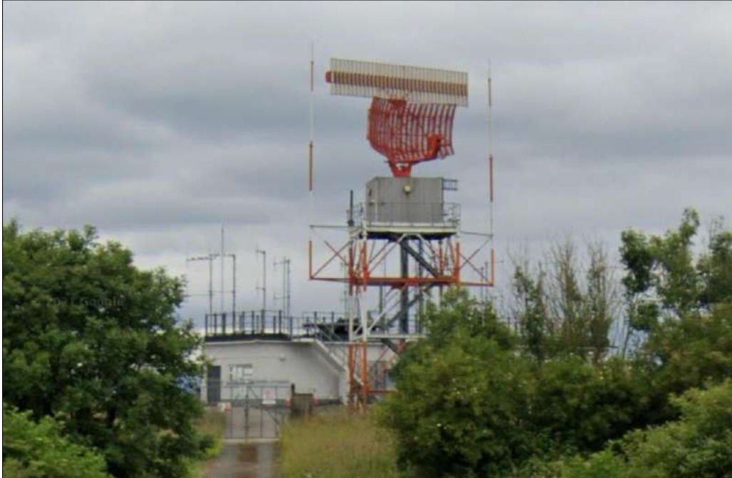
Figure 12. Dublin Airport MSSR Radar Station #1
