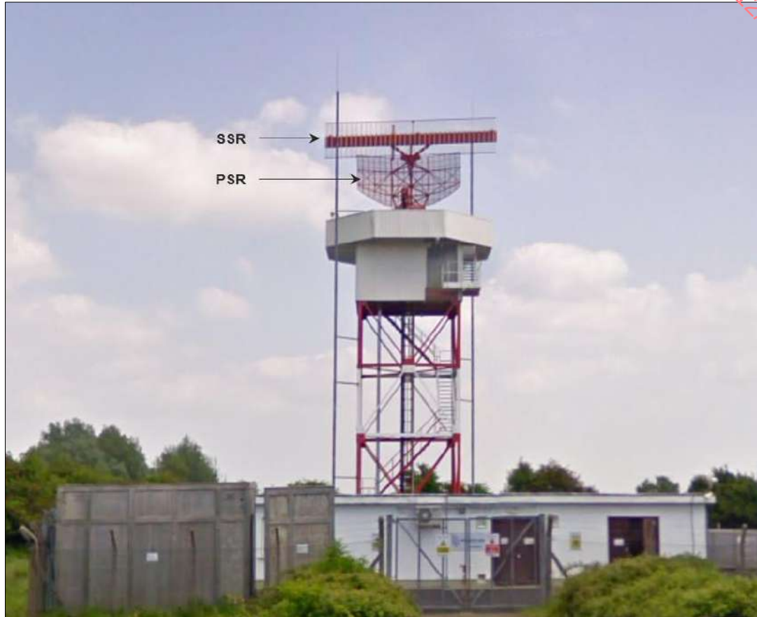
Figure 10. Shannon Airport Radar Station
